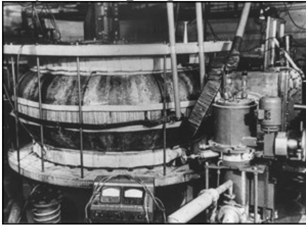
The world's first tokamak device: the Russian T1 Tokamak at the Kurchatov Institute in Moscow. Plasmas in the range of 0.4 cubic metres were produced in its copper vacuum vessel.
