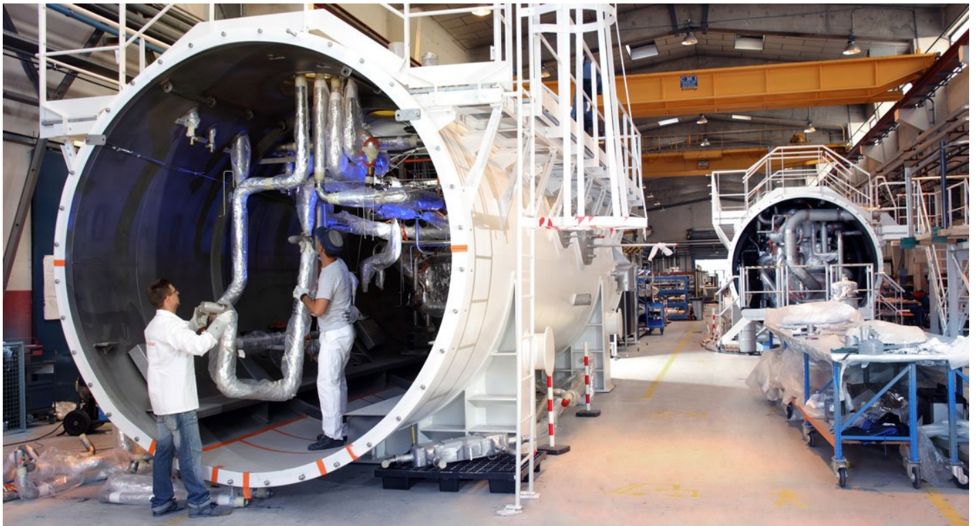
| The ITER Tokamak will rely on the largest cryogenic plant infrastructure ever built.
