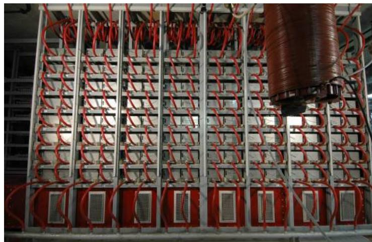
Figure 40 - Gyrotron main power supply installed at CRPP, Lausanne
