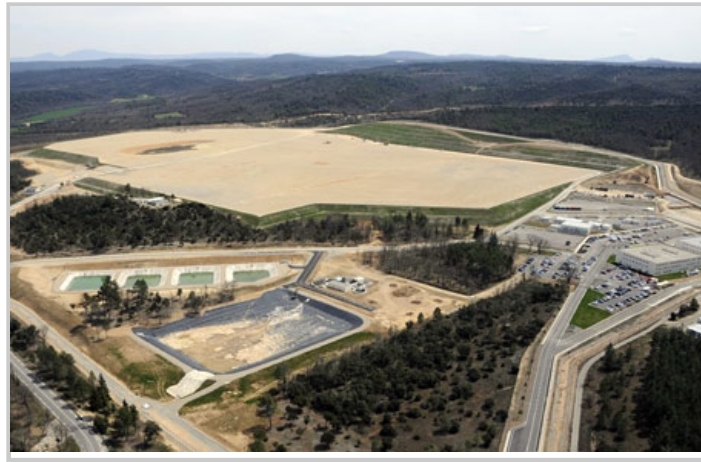
An aerial view of the ITER construction site in Cadarache, France, June 2010. (Courtesy: Agence ITER France)
