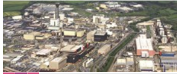
Sellafield Legacy Ponds Decommissioning
