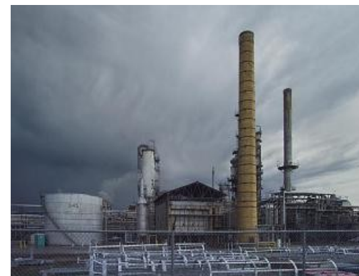
Coal Power Plant
