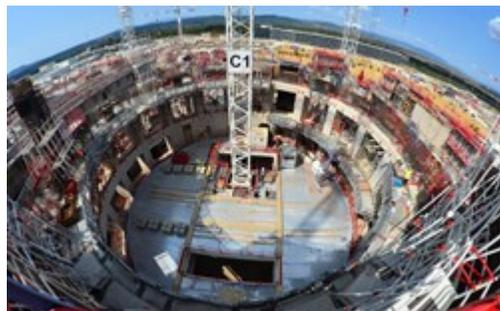
On a cleared, 42-hectare site in the south of France, building has been underway since 2010. The ground support structure and the seismic foundations of the ITER Tokamak are in place and work is underway on the Tokamak Complex—a suite of three buildings that will house the fusion experiments. Auxiliary plant buildings such as the ITER cryoplant, the radio frequency heating building, and facilities for cooling water, power conversion, and power supply are under construction.
