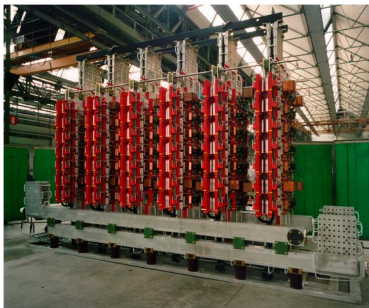
Fig. 6: 90 MVA main converter prototype built and tested in 1998
