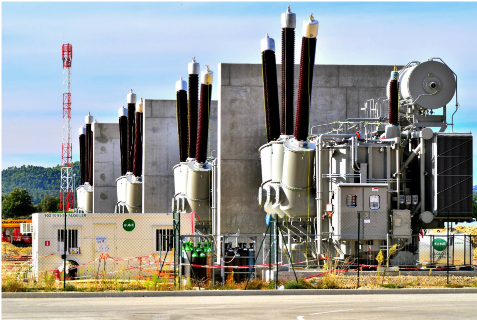
PPPL procured and shipped four massive transformers from Hyundai Industries in South Korea to ITER as part of the SSEN Project. Photo courtesy of © ITER Organization
