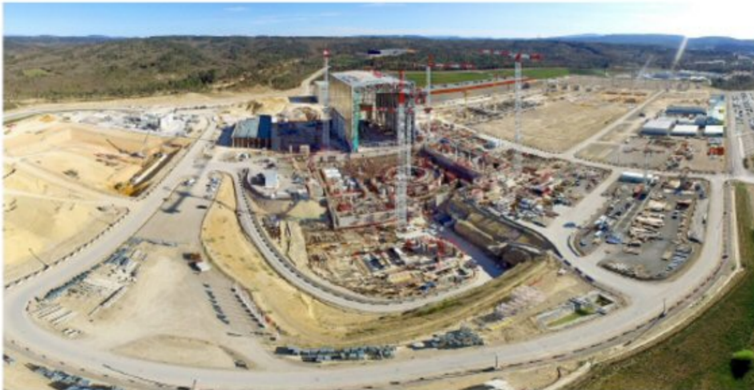
ITER work site-April 2016
