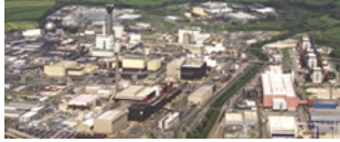
Sellafield Legacy Ponds Decommissioning
