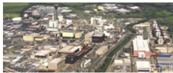
Sellafield Legacy Ponds Decommissioning
